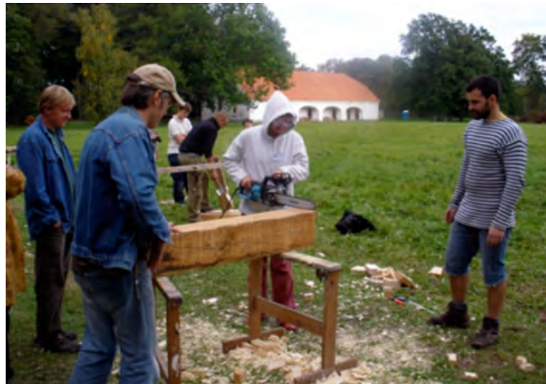
Figure 3.24. Here we are cutting out the splice with a chainsaw. Tarmo Tammekivi ( far right ) is supervising the amateurs.
