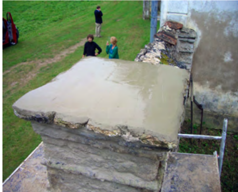
Figure 2.15. The broken flagstones on top of garden posts A and B had to be replaced with a topping of cement mortar because similar new stones were not available.
