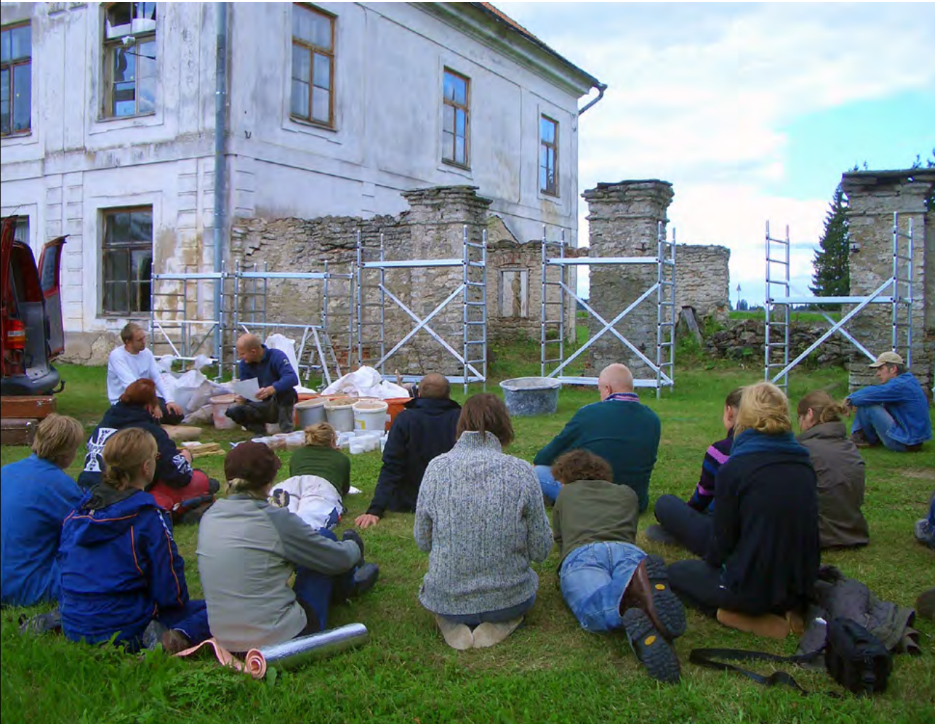
Figure 2.1. Students learning about mortars and restoration of stone walls. Teachers Taavi Leis ( left ) and Kermo Jürmann introduce correct materials and tools. Gateposts which are to be restored stand in the background waiting for their restorers. From left: gatepost A (Swedish students), B (Finnish students) and C (Estonian students).
