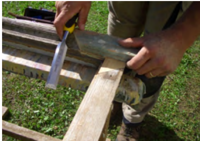
Figure 3.37. A new piece of wood has replaced an old decayed part.
