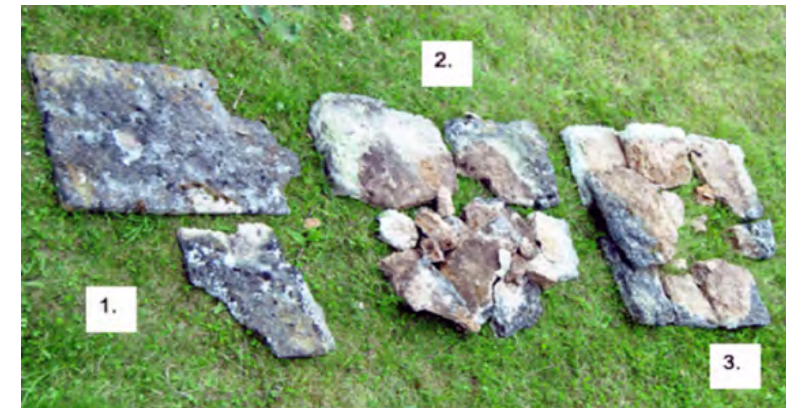
Figure 2.14. Dismantled stones from gatepost: top level (1), second layer (2)—middle part, and right—third layer from top, bottom part of gatepost profile (3).
