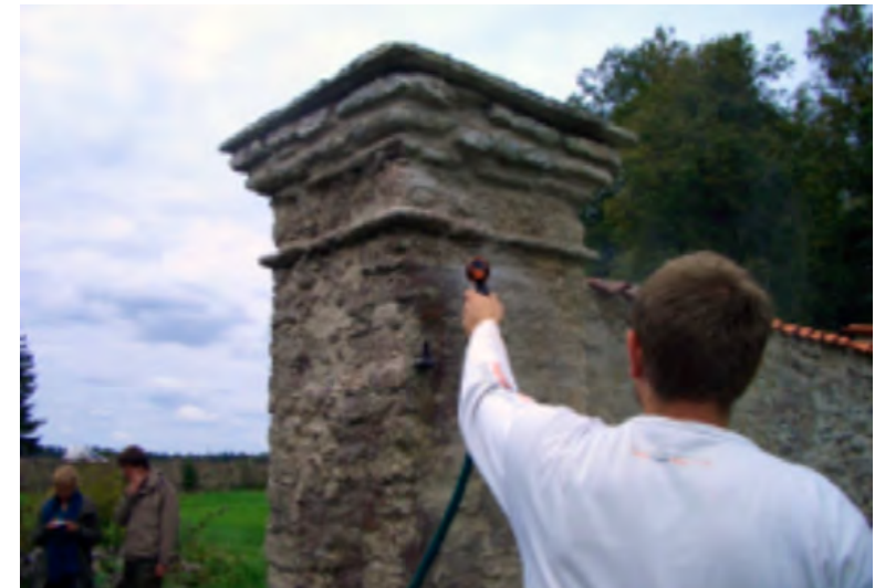
Figures 2.16–17. Finishing touches are being applied on gatepost C.
