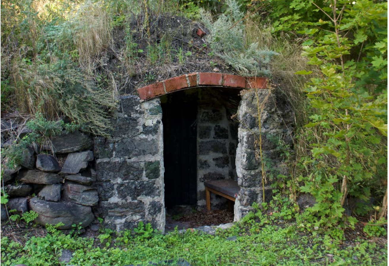
FIGURE 1.5. An old disused root cellar built into a slope. Photograph by Towe Andersson.
