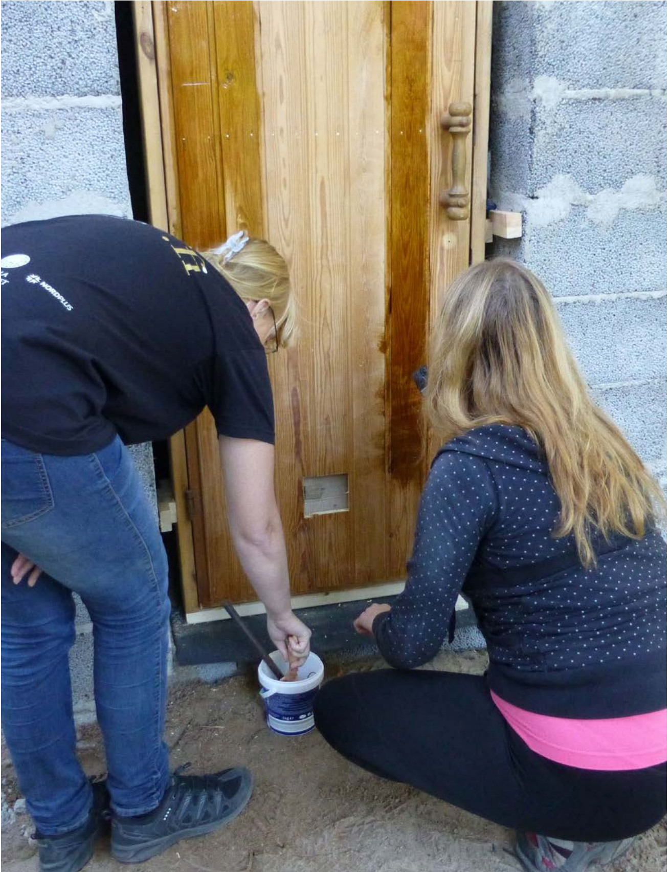
FIGURE 4.7. A mixture of tar, boiled linseed oil and turpentine was applied on the outside of the front door. Photograph by Kirsti Horn.
