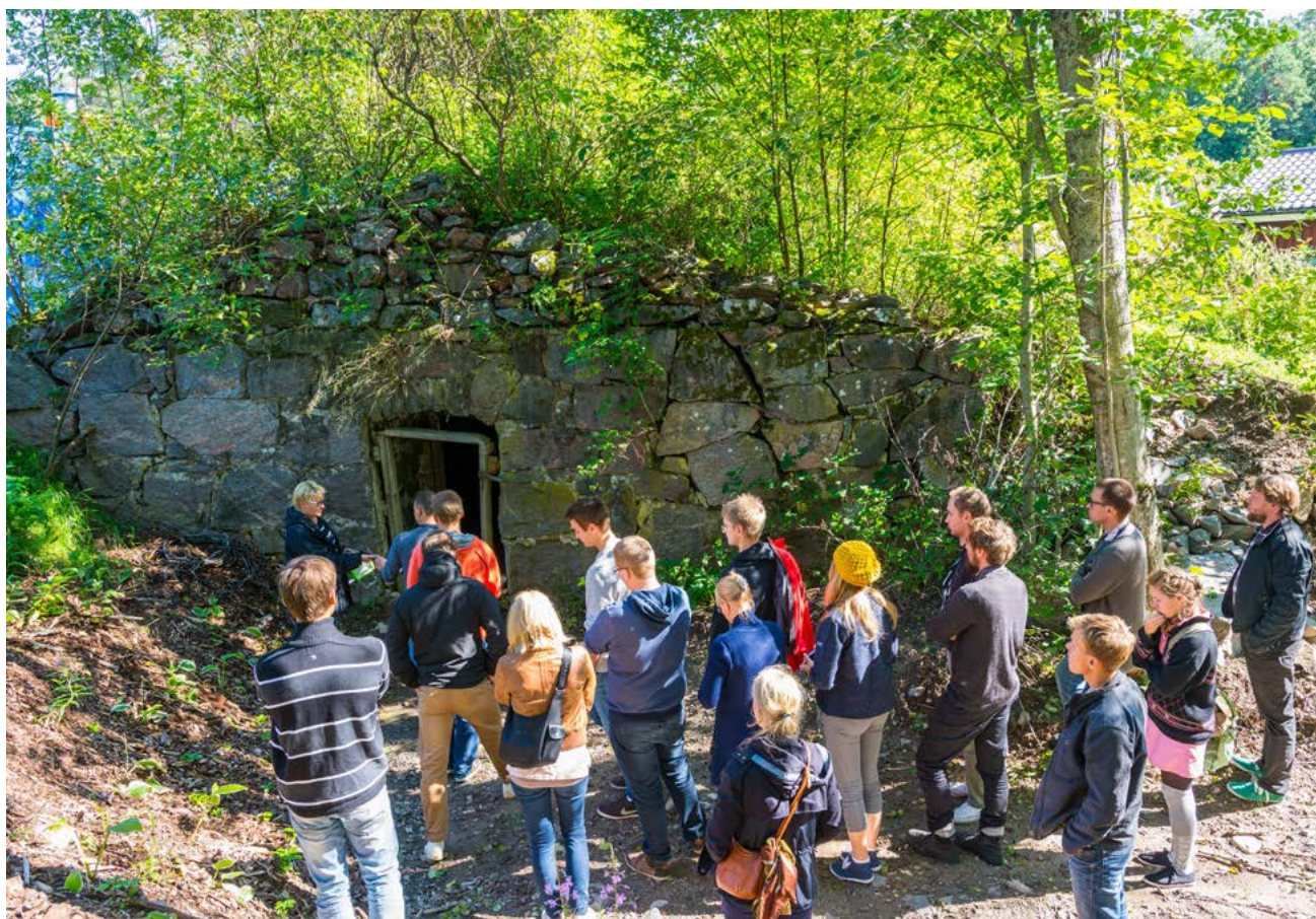
FIGURE 1.1. The historic root cellar of a grand scale built of granite at Västankvarn experimental farm, Finland, was presented by Ulrika Grönvik to the authors of this report. Note the thickness of the double skin masonry in the entrance. Photograph by Towe Andersson.
