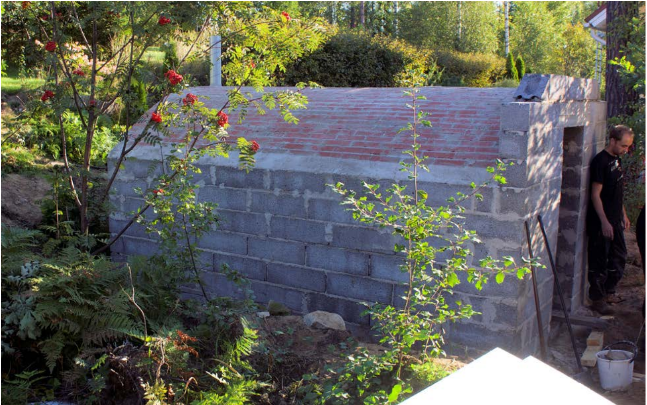
FIGURE 1.4. Model root cellar (before damp proofing) built by students at Novia and participants to the intensive course in Ekenäs, Finland in the autumn of 2014. Photograph by Towe Andersson.
