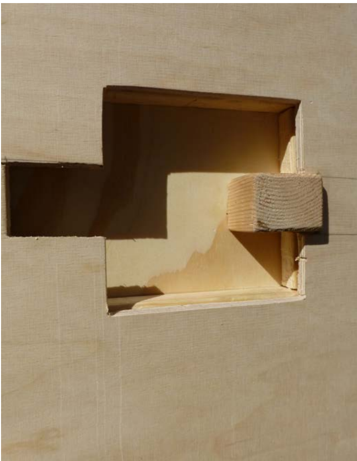
FIGURE 4.3. The sliding air vent hatch. Photograph by Kirsti Horn.
