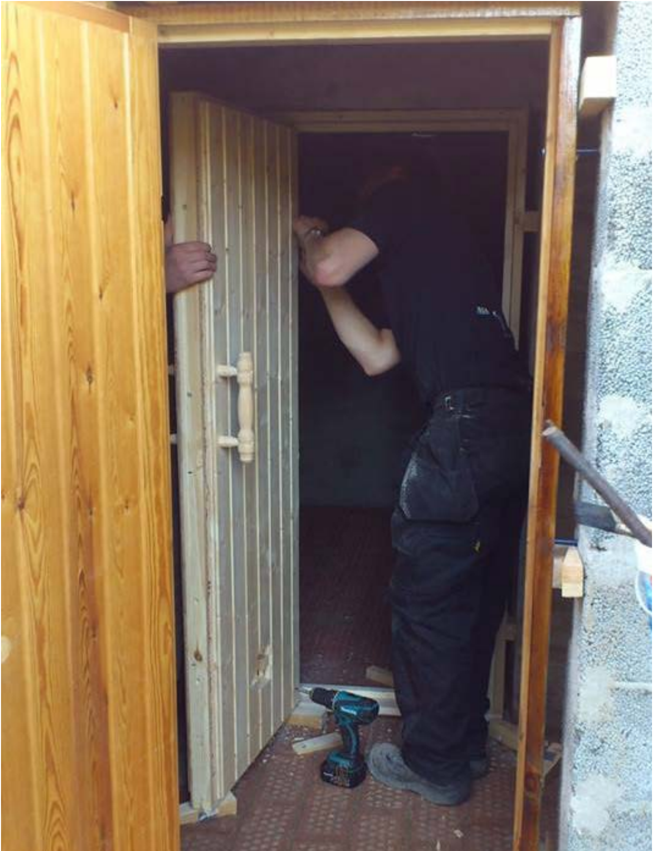
FIGURE 4.6. Doors are being mounted. Photograph by Sanna Svensson.
