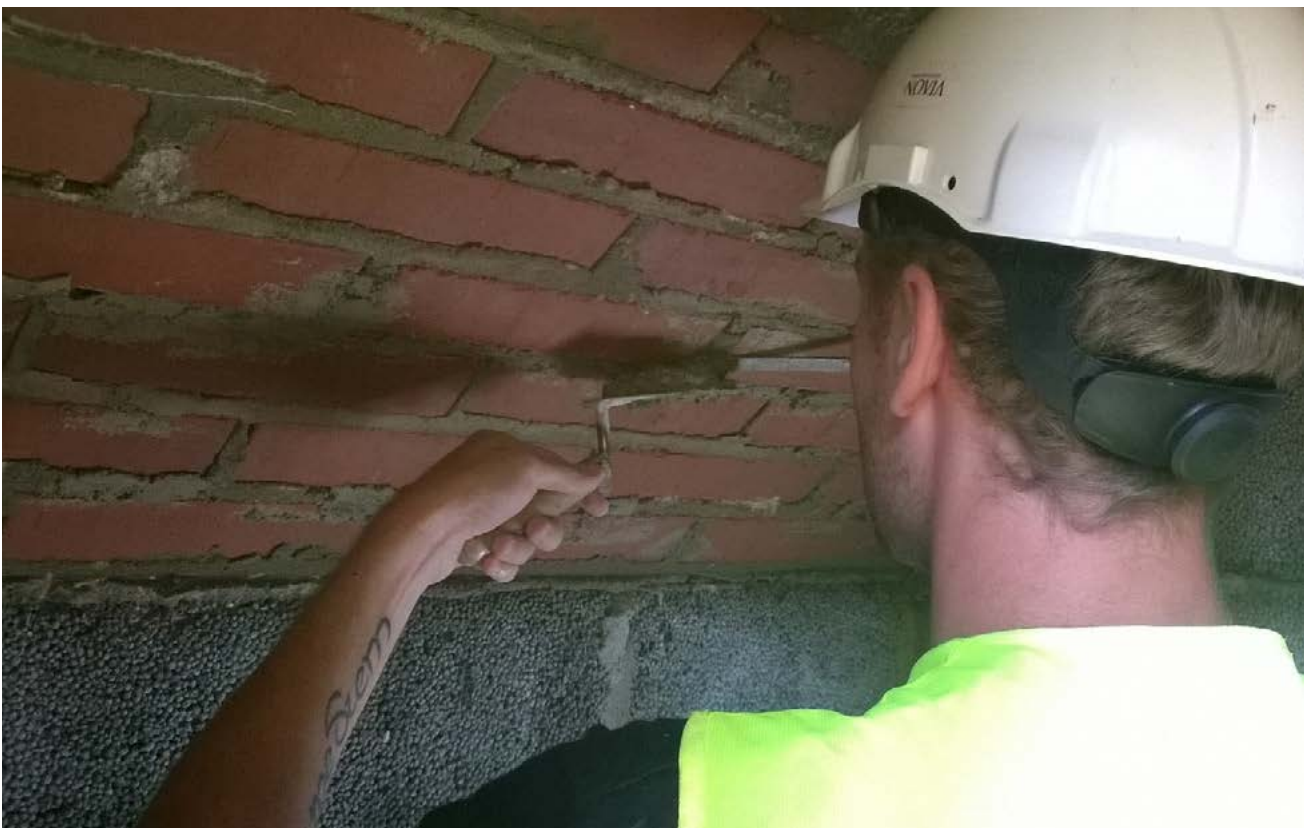
FIGURE 2.20. The biggest cavities were filled. Photograph by Kirsti Horn.
