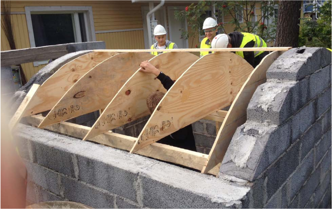
FIGURE 2.13. The rounded sheets of plywood must stay straight to give a perfect, symmetrical shape. Photograph by Sanna Svensson.
