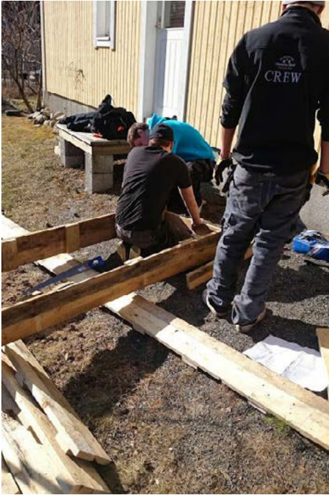
FIGURE 2.4. The formwork for the plinth was built of boards. Photograph by Niklas Nyman.
