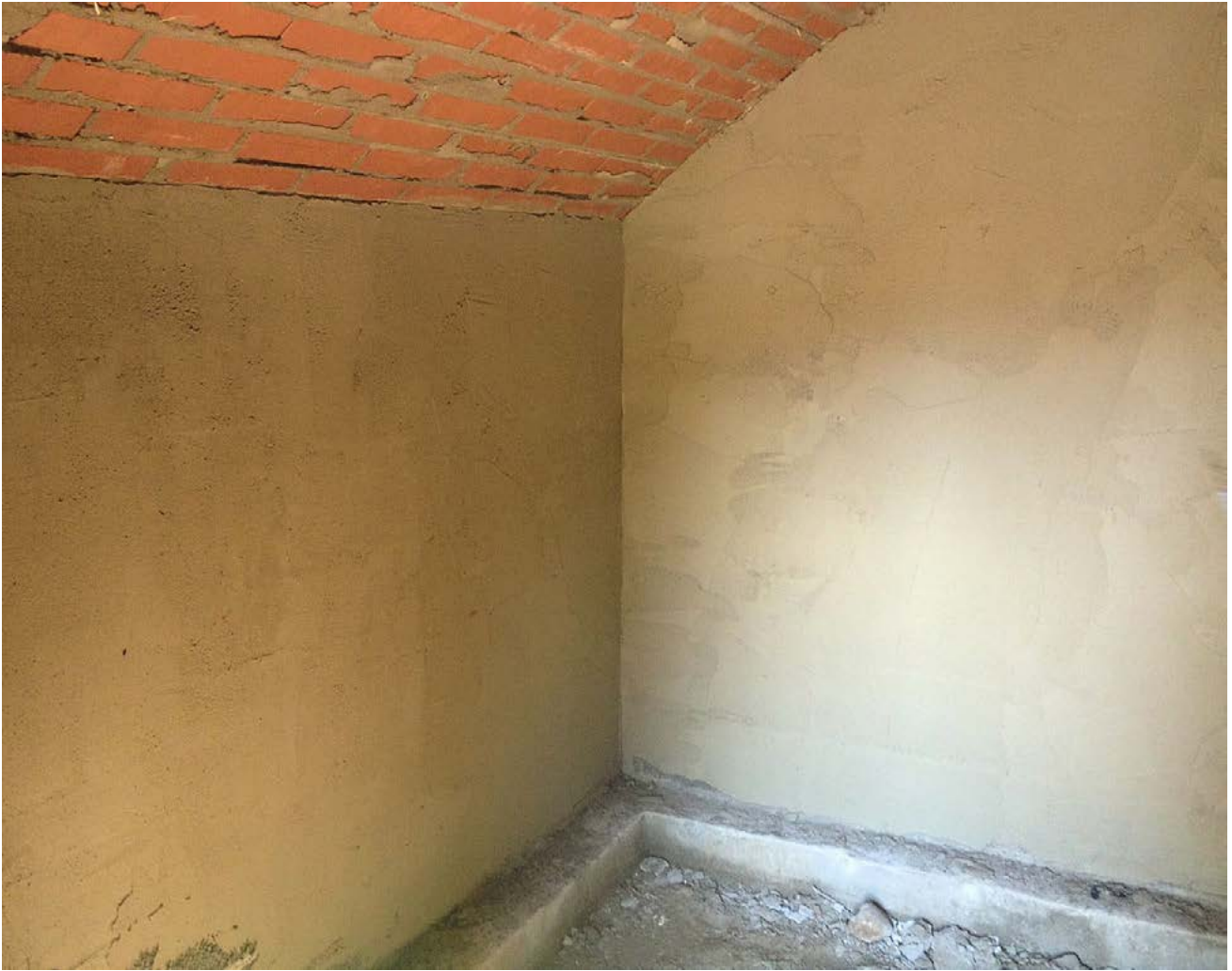
FIGURE 3.3. Plastering almost completed. Photograph by Sanna Svensson.
