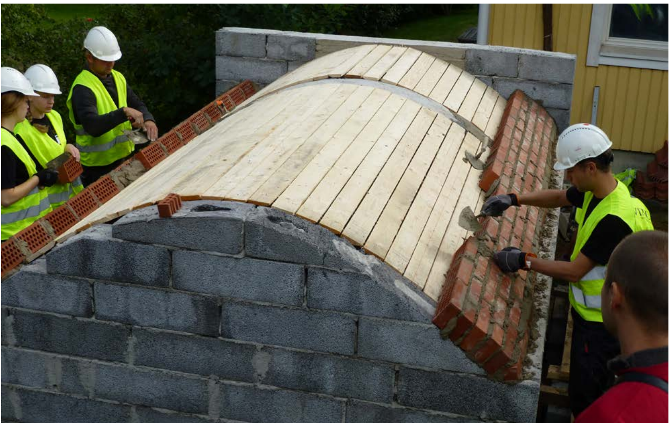
FIGURE 2.18. Bricks are laid from both sides of the barrel shaped centering. Photograph by Kirsti Horn.
