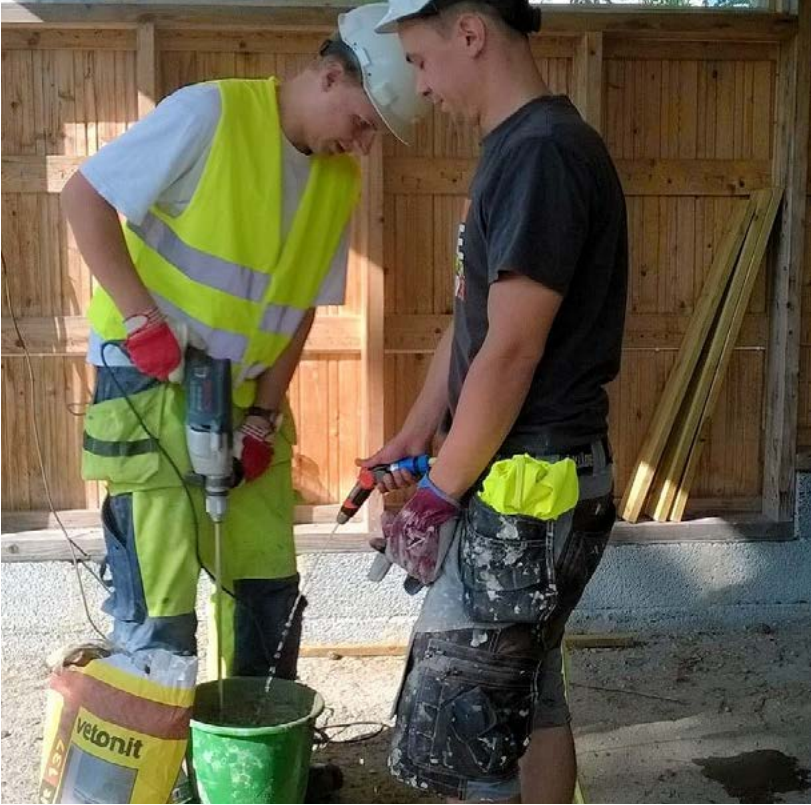
FIGURE 3.1. Students are mixing the plaster with an electric plaster mixer. Photograph by Kirsti Horn.
